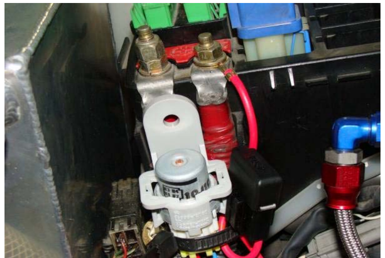
Example of the Relay Mounting.
